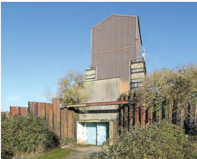
The present entrance to P2 was the original exhaust gas outlet
